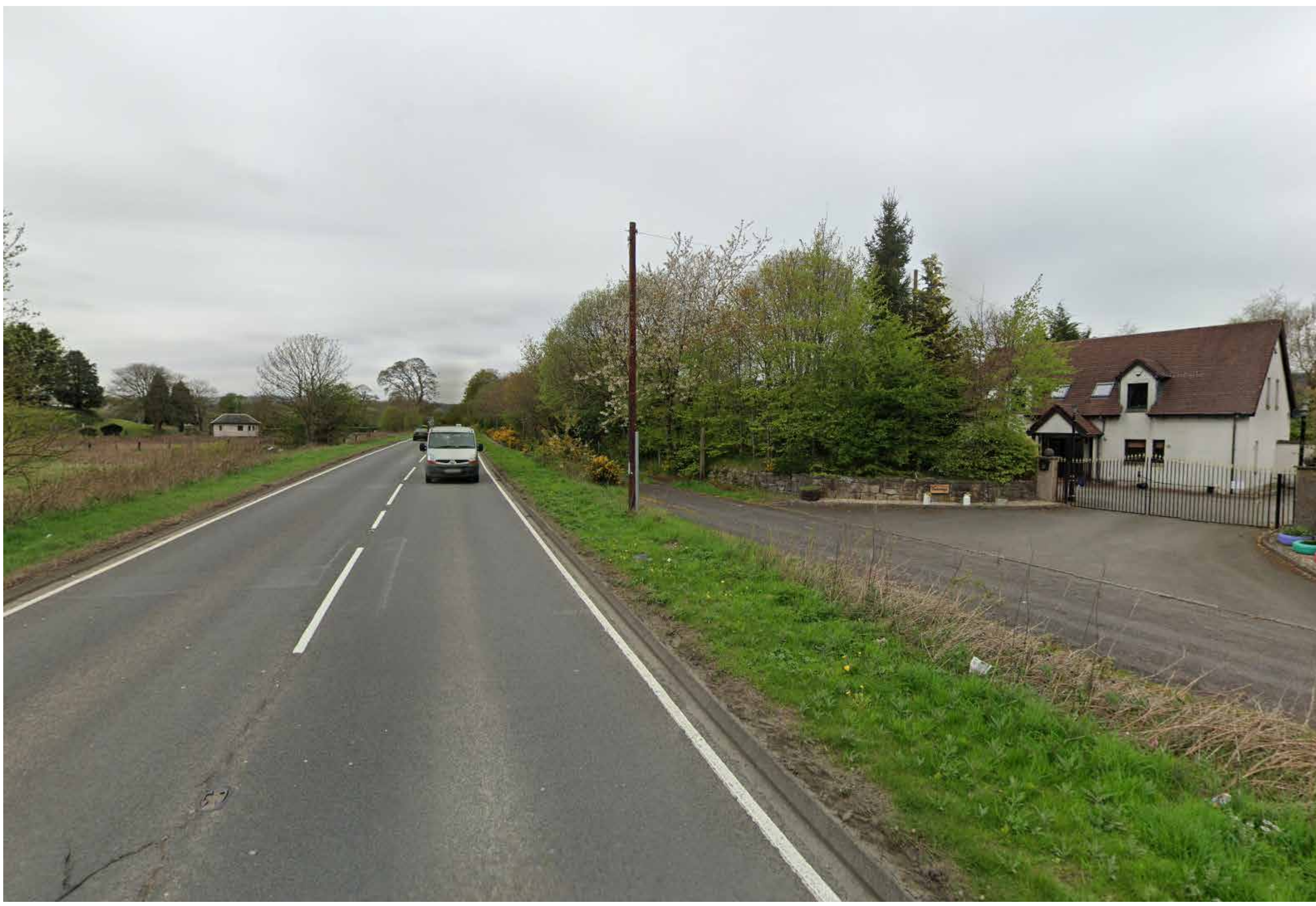
4. View north-west along A883
